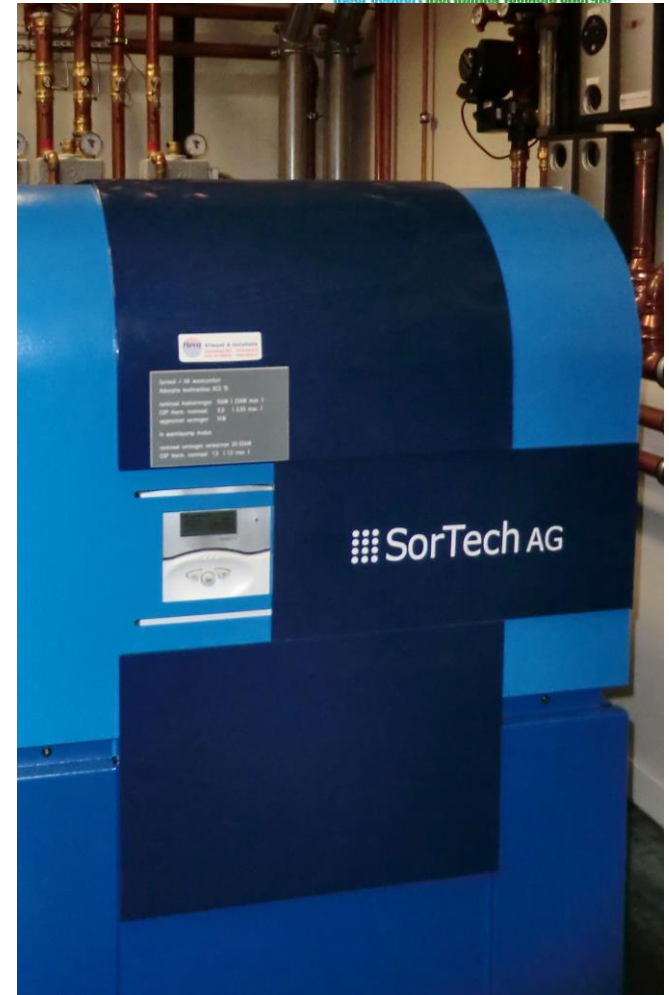
Adsorption heat pump
